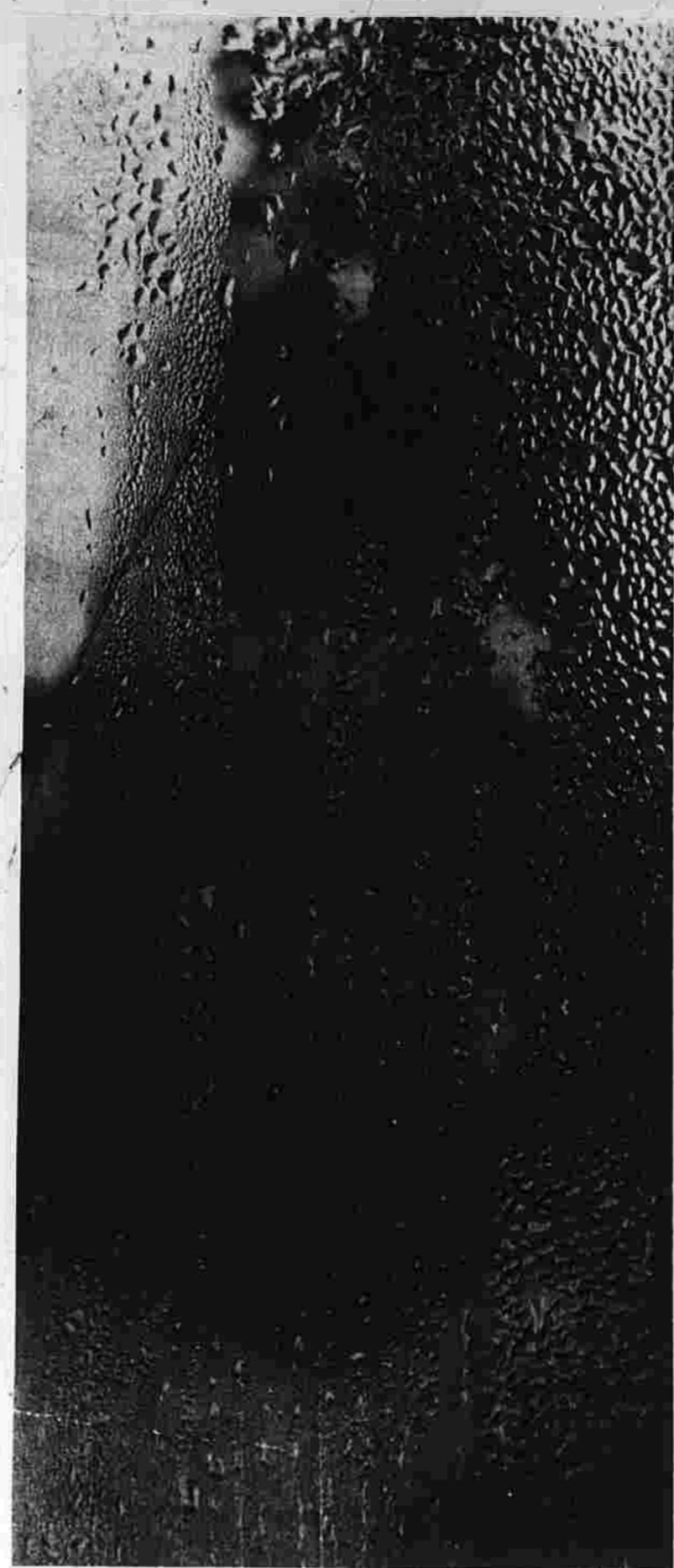
Moisture on glass (inside)
